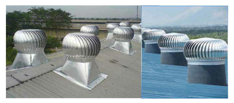
Turbine Ventilator is air circulation control tool that use to suck out hot air, dust, and smoke from inside the room withot using any electrical power. Which means this technology is clean, efficient, and free!
